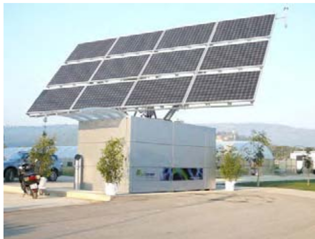
Fig. 3: Solar filling station for electric vehicles at the Castello Monte Vibiano Wine and Olive farm.
