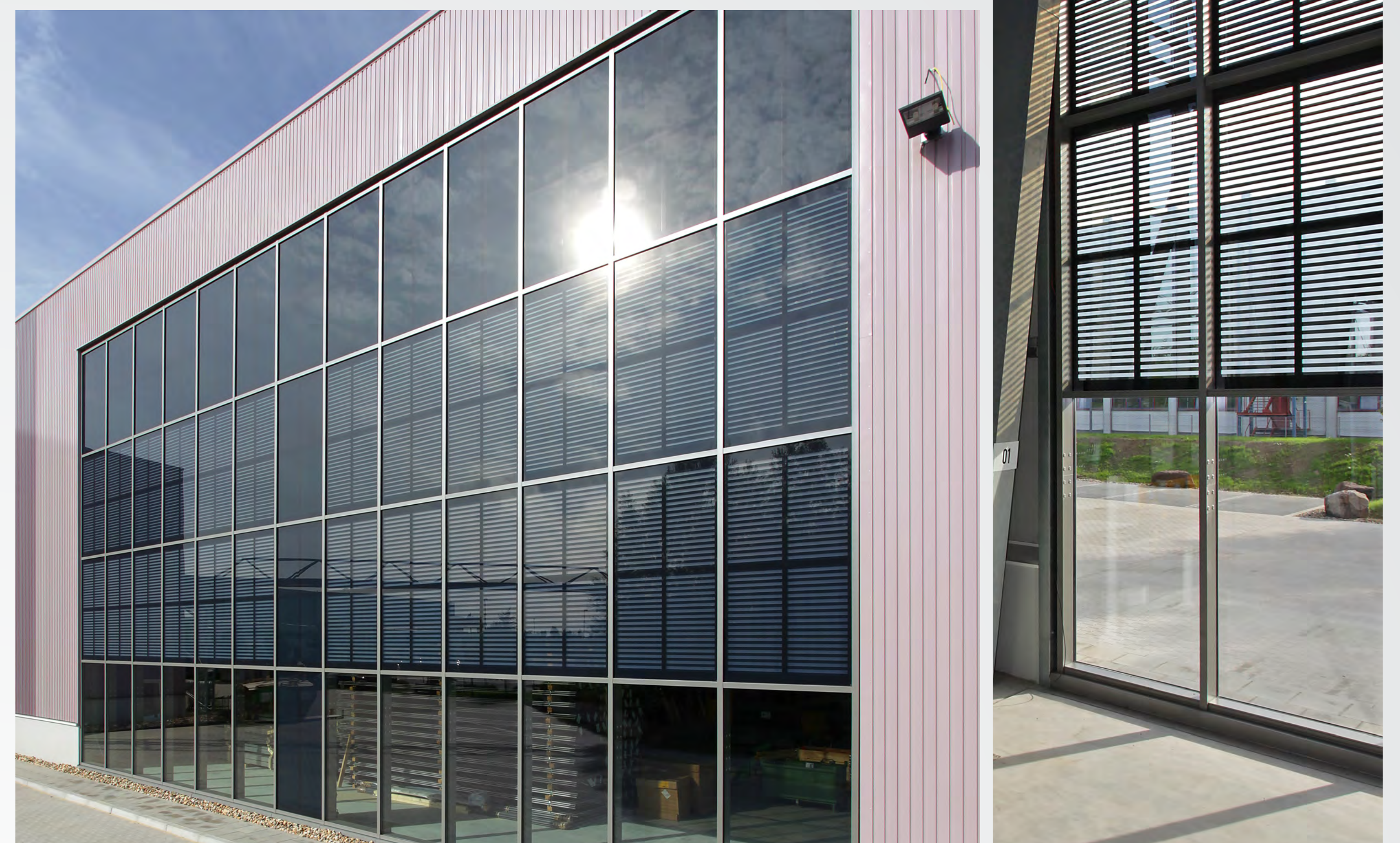
Fig. 3: RP Technik BIPV Steel Façade system (Source: RP Technik GmbH Profilsysteme)
