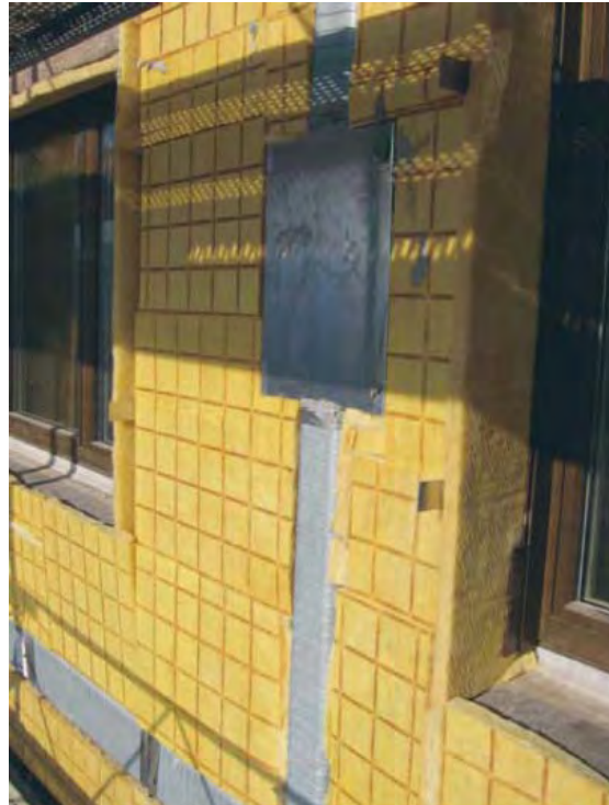
Section trough the facade with flat ducts integrated in the heat insulation (S+P-Haustechnik)
