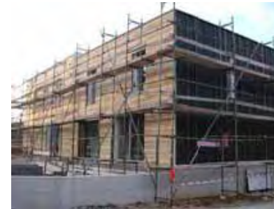
Mounting of the wind-tight layer, of the substructure for the ventilated cladding and of the cladding
