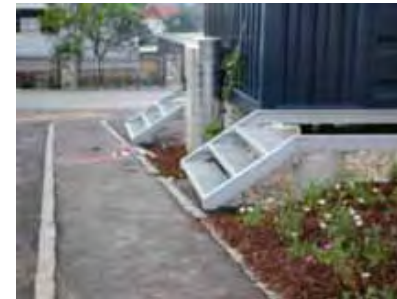
Positioning of the storage container and of the air inlet for the ventilation system; mounting of the entrance stairs
