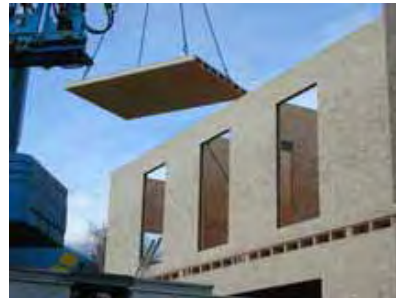
Mounting of the prefabricated walls, the ceiling and the roof elements (OSB 8000)
