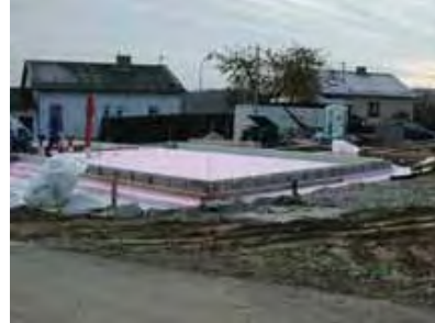
Building the floor slab on the heat insulation
