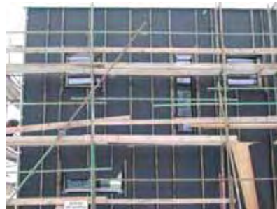
Mounting of the wind-tight layer, of the substructure for the ventilated cladding and of the cladding
