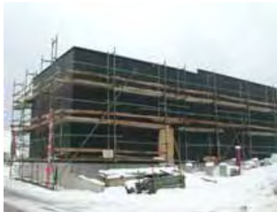
Mounting of the wind-tight layer, of the substructure for the ventilated cladding and of the cladding
