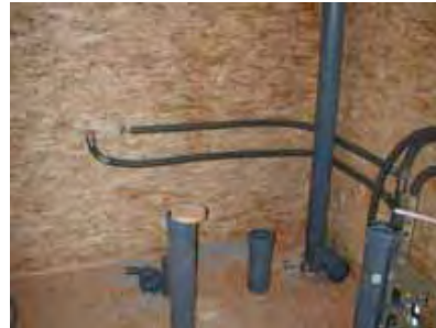
Mounting of the ventilation ducts and the installation pipes; “Blower door test”
