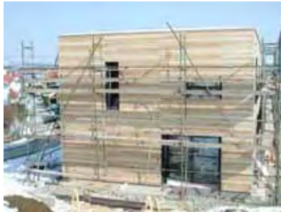
Mounting of the wooden cladding
