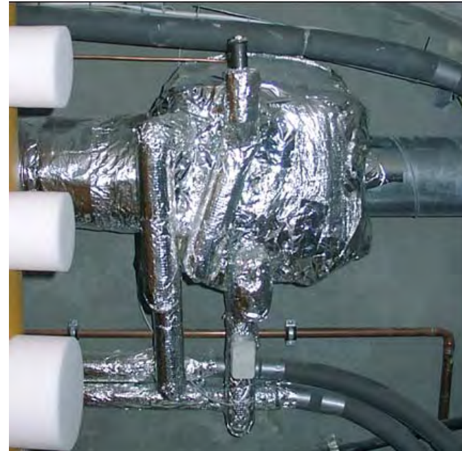
Post-heater in the inflow pipeline (before and after the addition of insulation)
