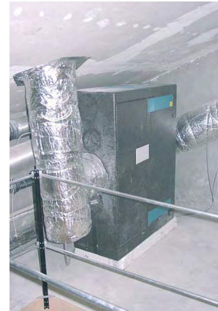
Ventilation unit with heat exchanger in the building services floor
