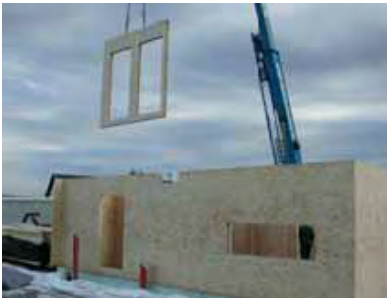
Mounting of the prefabricated walls, the ceiling and the roof elements (OSB 8000)
