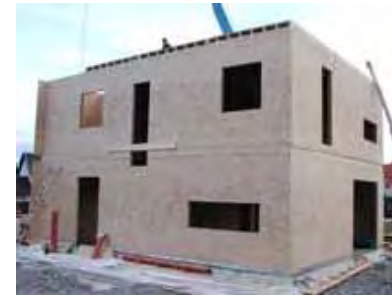
Mounting of the prefabricated walls, the ceiling and the roof elements (OSB 8000)
