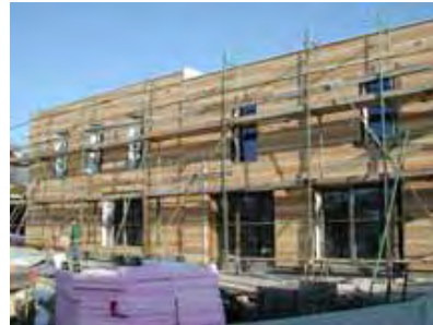
Mounting of the wooden cladding
