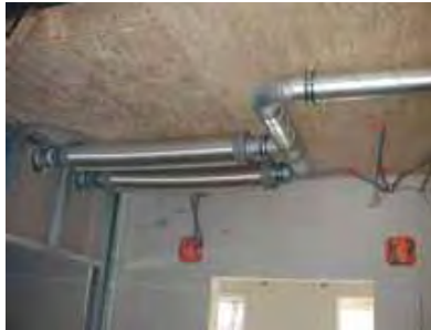
Mounting of the ventilation ducts and the installation pipes; “Blower door test”
