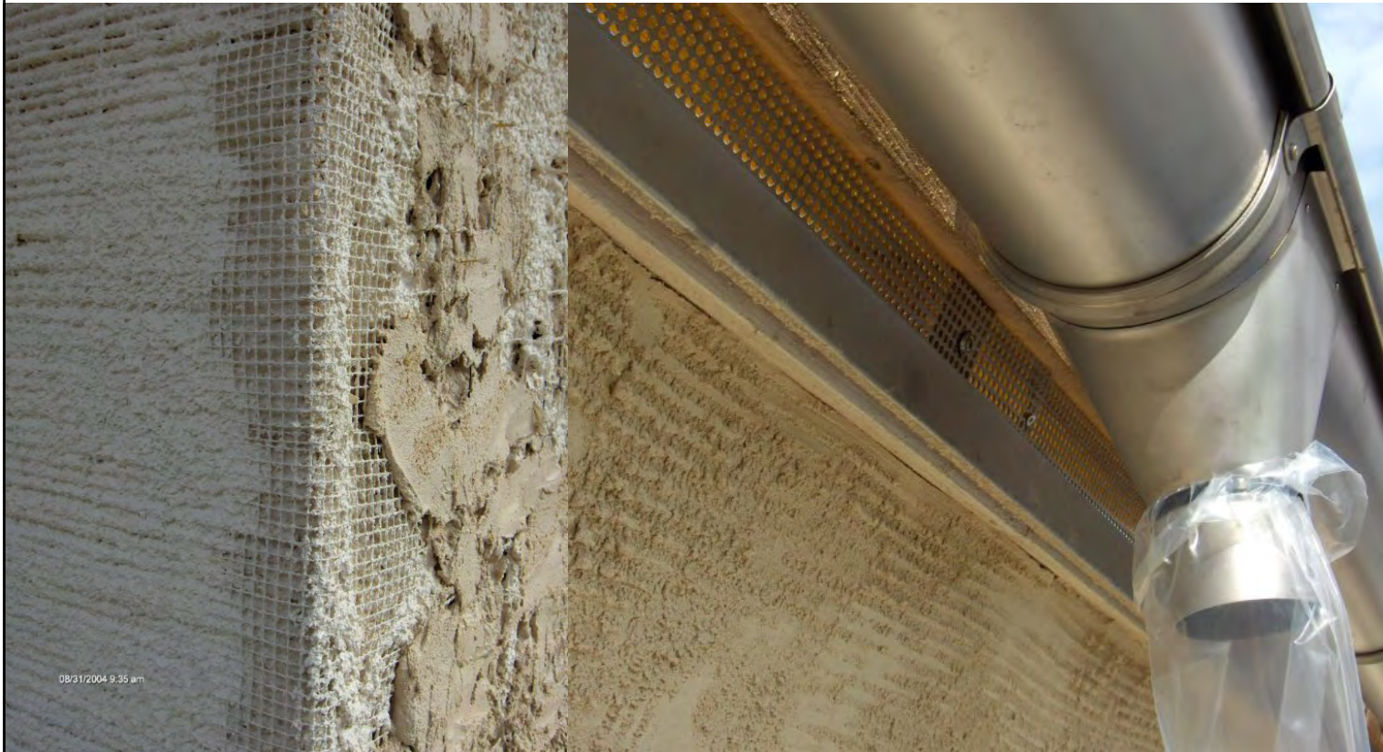
Spray on the loam plaster outside
