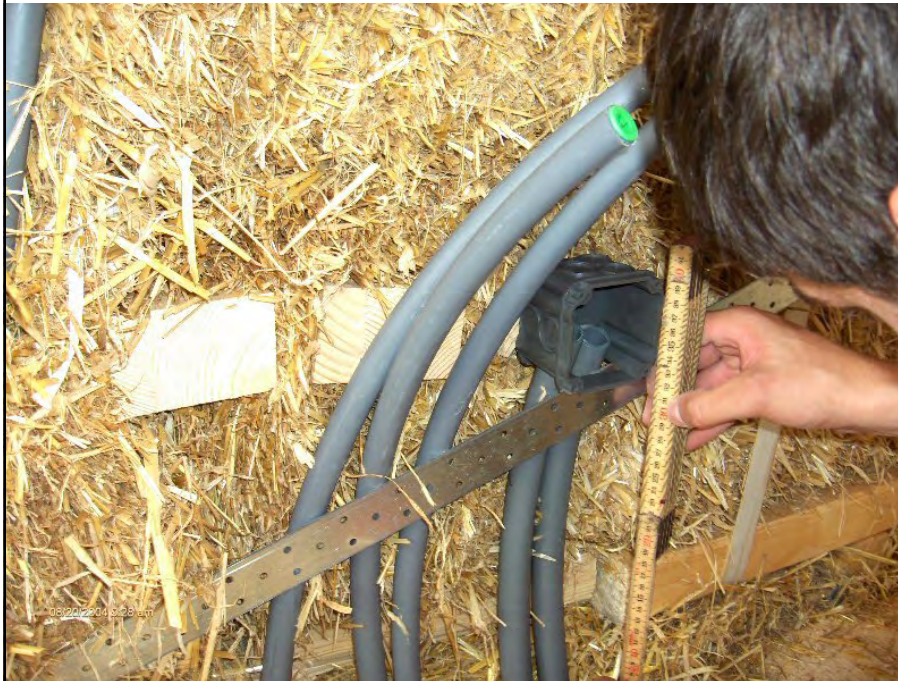
Mounting of the electrical installation
