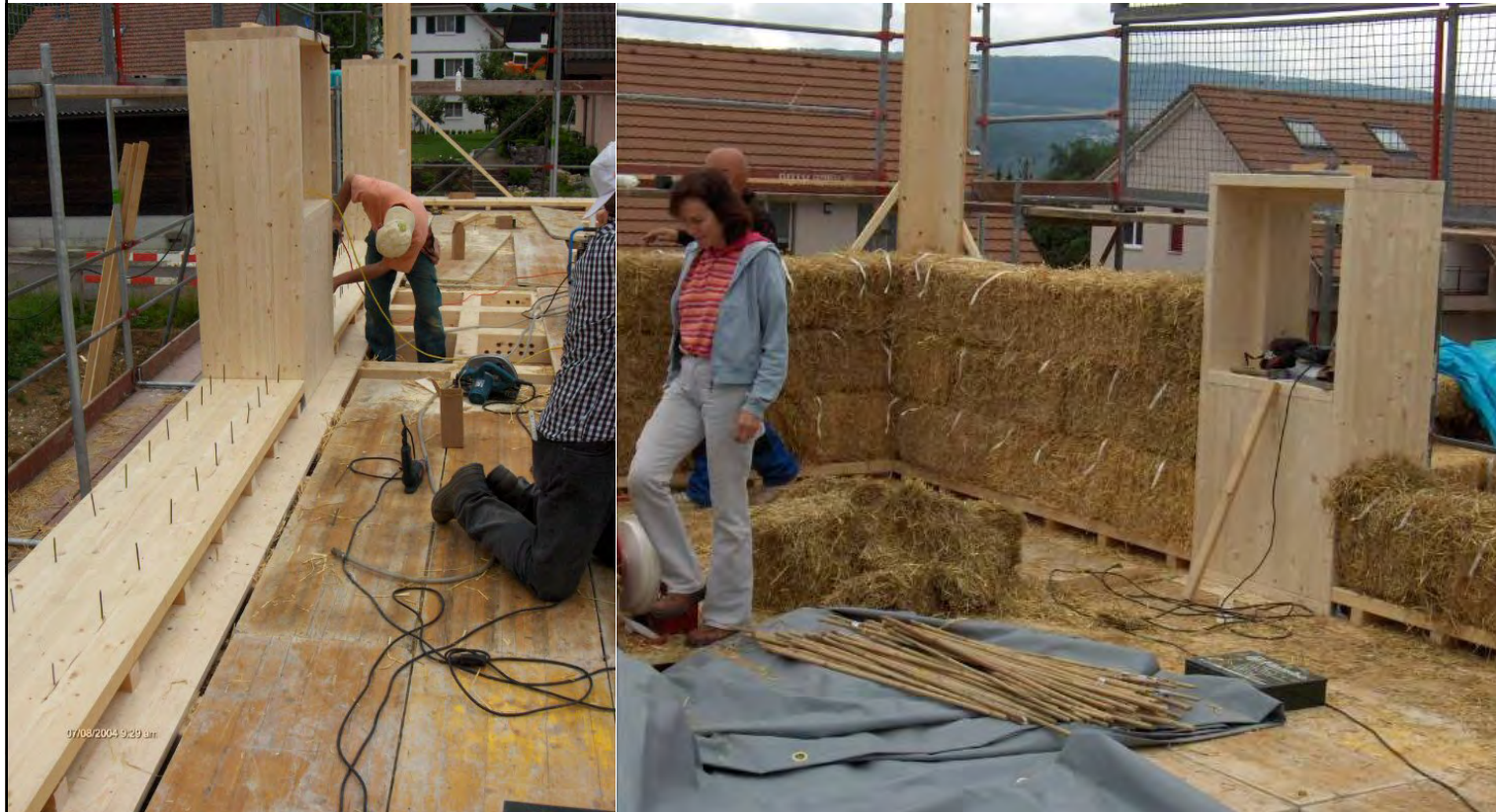
Outside wall construction of the upper floor
