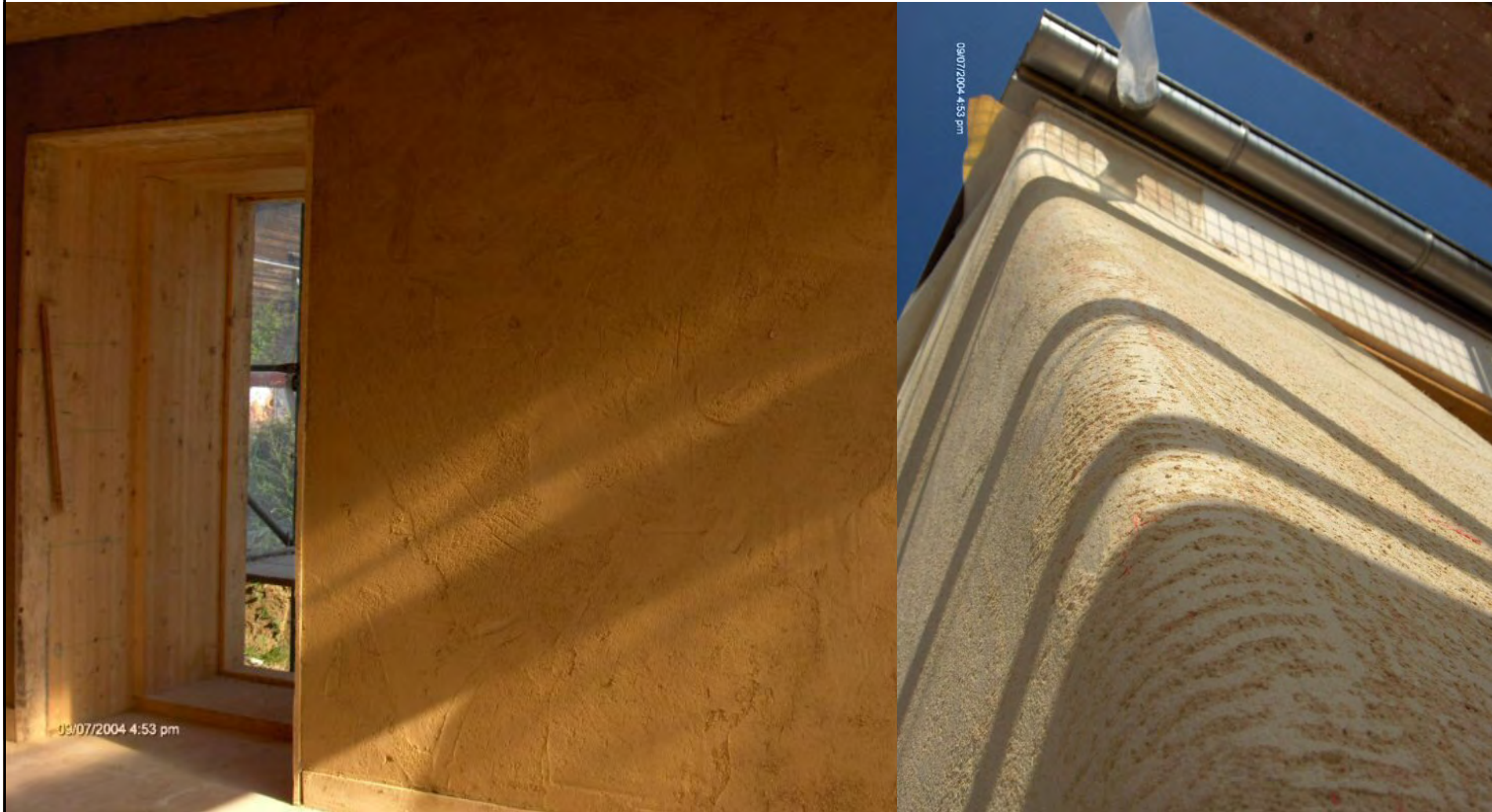
The finished inside and outside plaster
