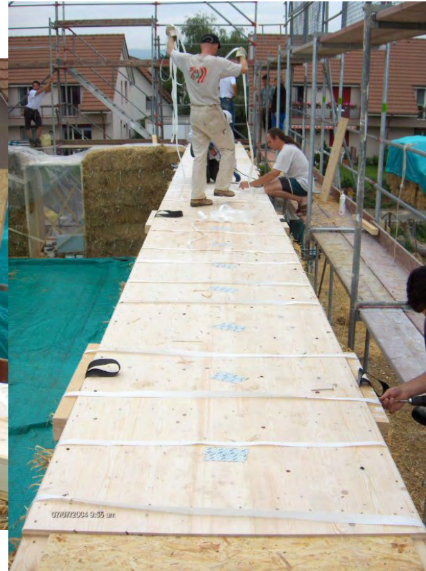
Clamping belts over the cover ring
