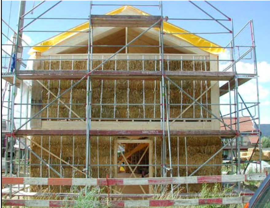
Preparation for outside plaster
