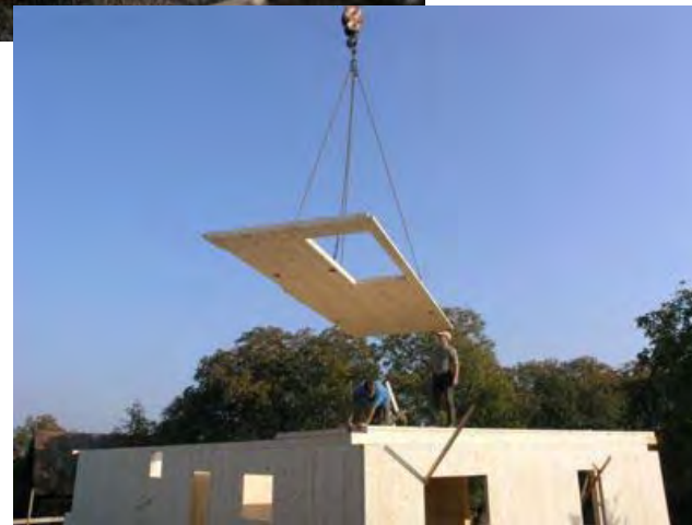
Fixing the ceiling with the aid of an crane.
