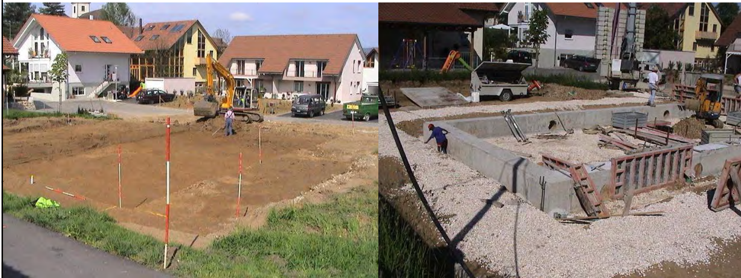
Excavation work and building the strip foundations.
