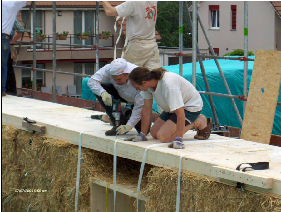
Bolting the laminated wooden cover belt
