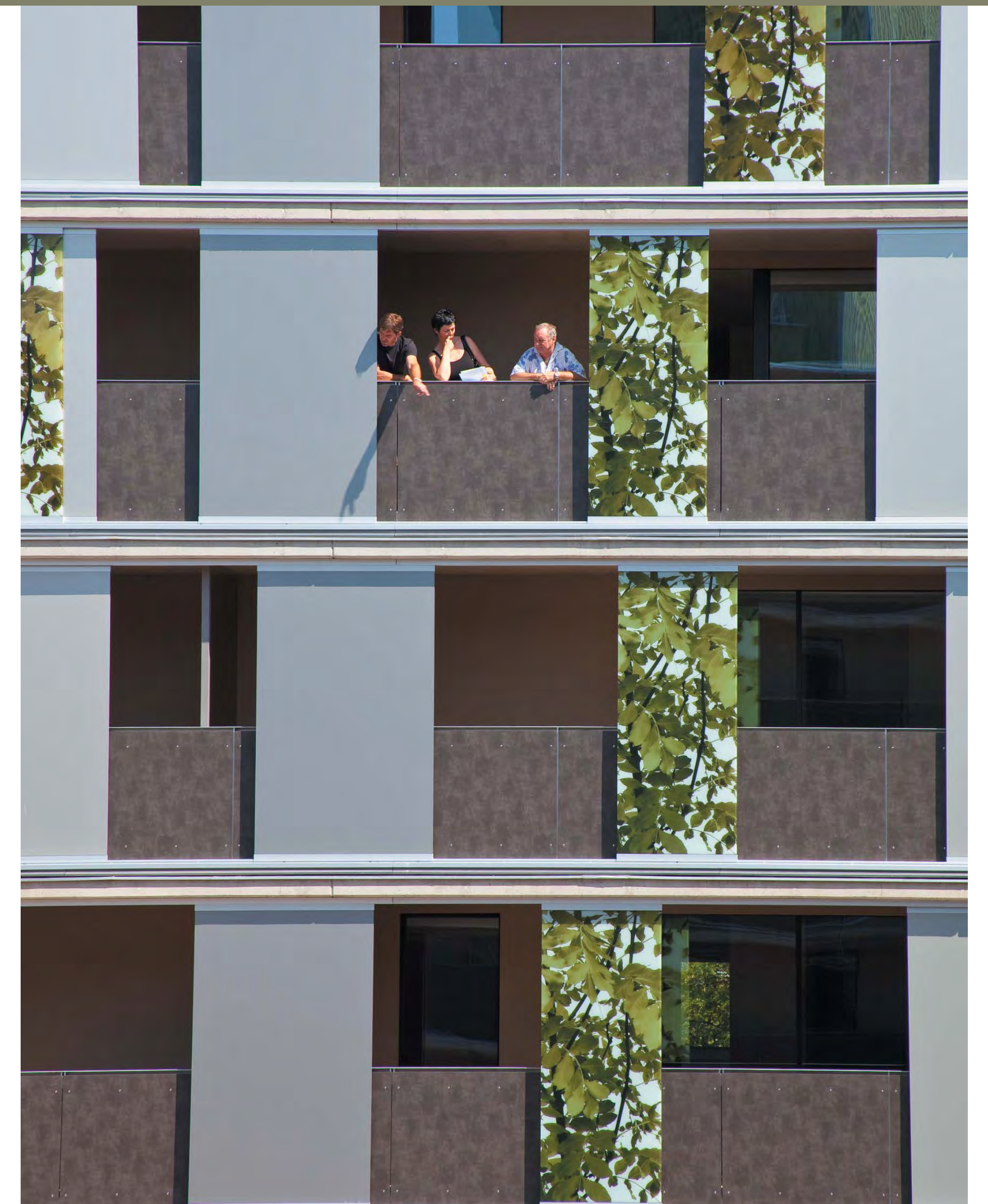
Fassade B2 | Facade B2
