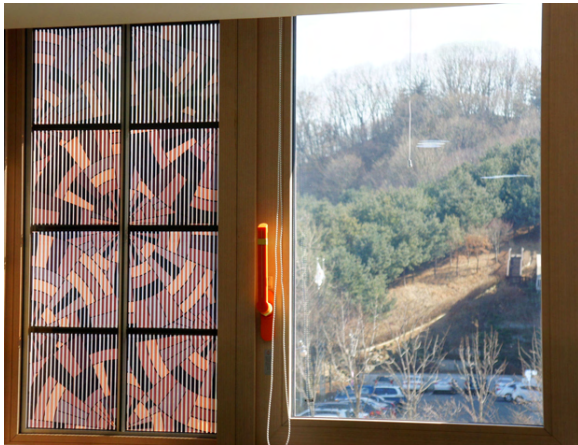
Abbildung 44: DSC window © Dyesol
