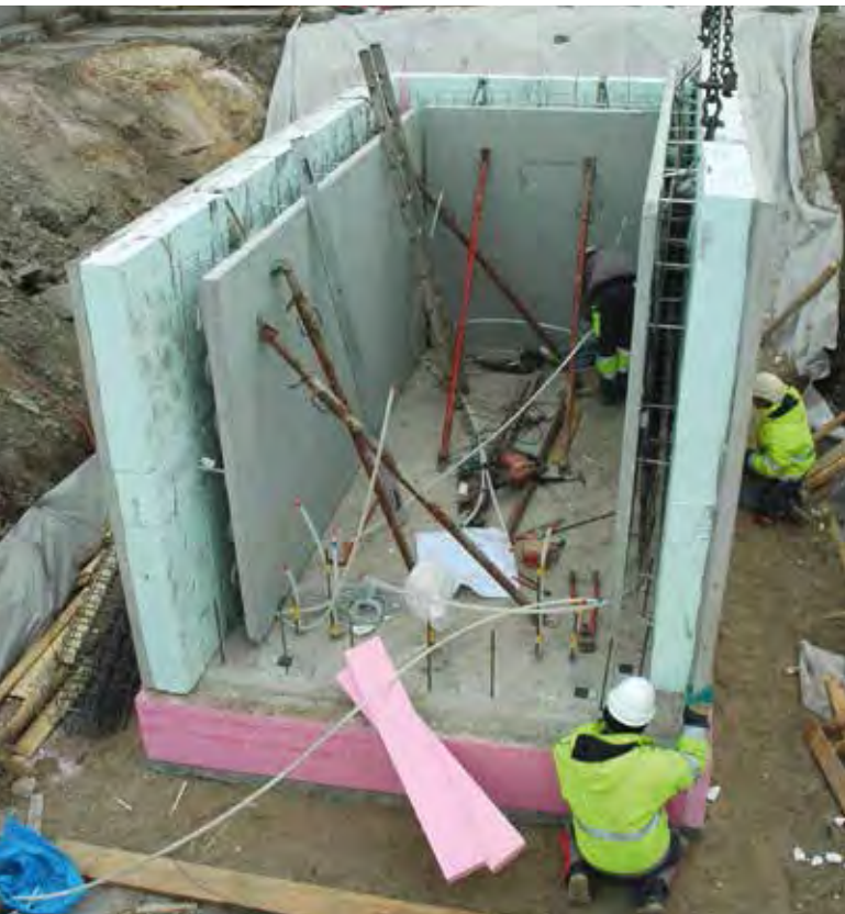
Abb. 5: Bauphase Keller 2, © VÖB/MABA/Oberndorfer/Trepka
